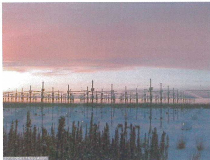
The HAARP-antenna array at Anchorage, Alaska 115
